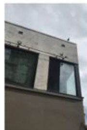
Soho club extension removed and replaced with modern loggia
