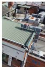
Roof plant units removed and replaced with a covered timber diagrid
