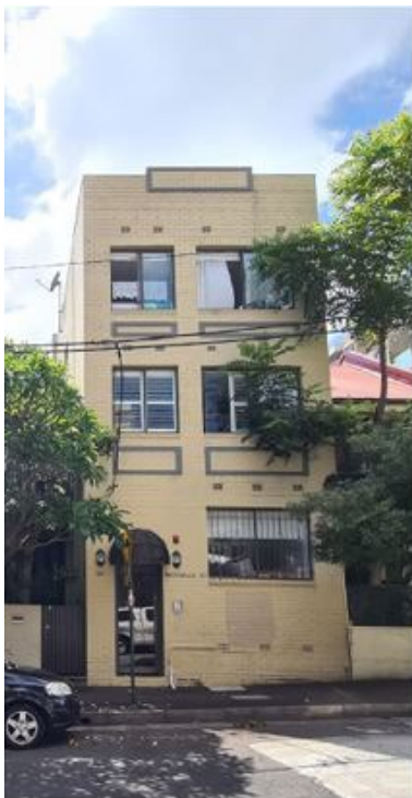
Image of 96 Brougham Street, showing the 1930s brick renovation which will be removed
