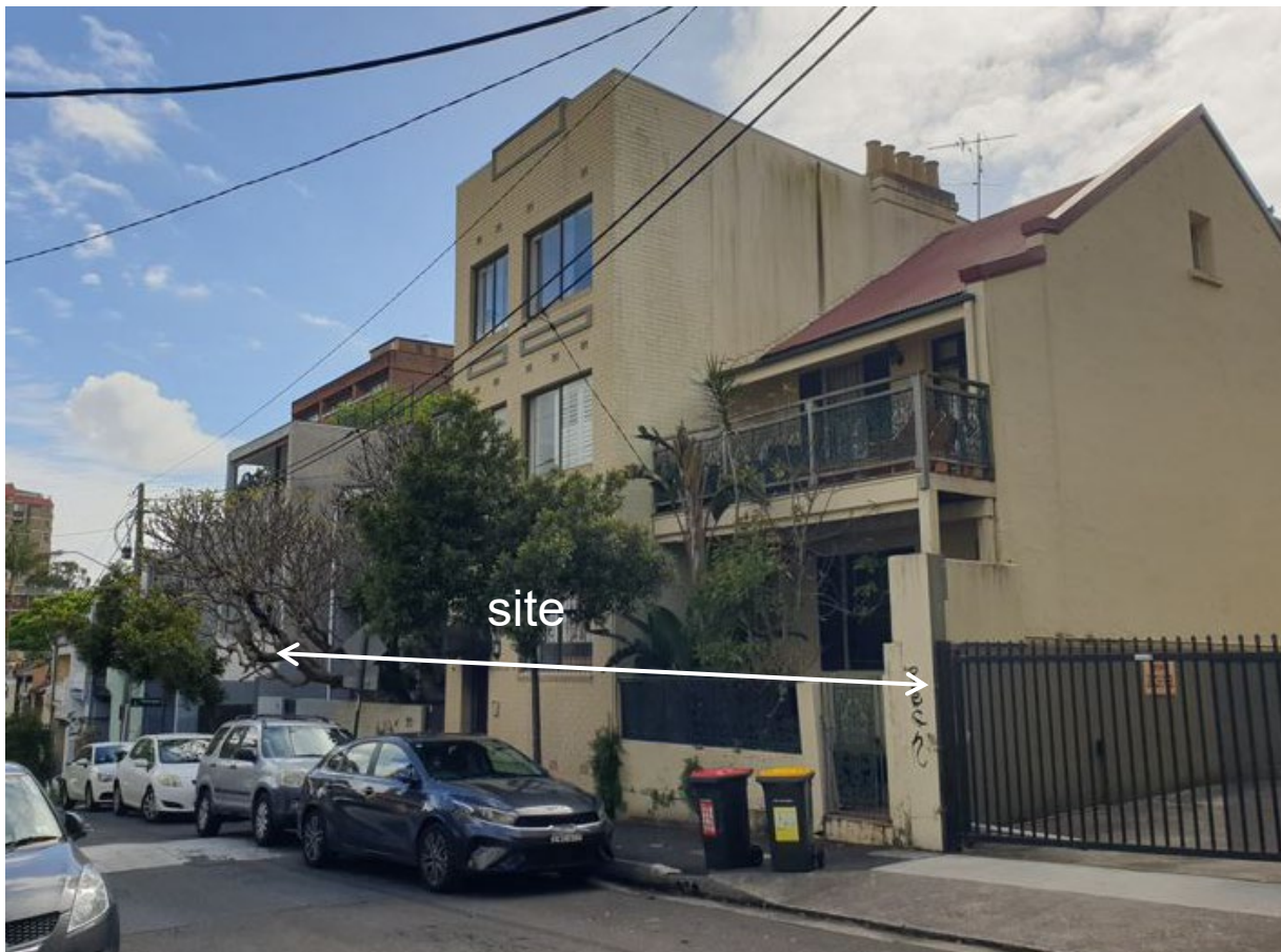
looking north along Brougham Street
